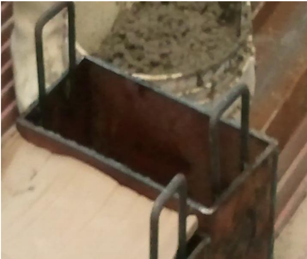
Figure 2: the beam B1(t6) is ready for concrete pouring.
